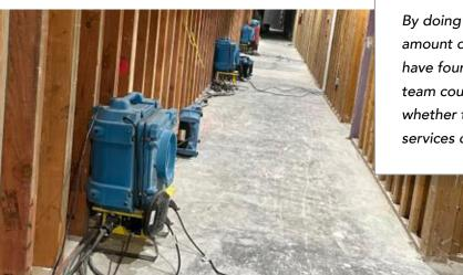
By doing a simple calculation, the team could determine the amount of air scrubbing and negative pressure needed to have four air changes per hour. From there, the restoration team could make their way through the building, determining whether the area required full demolition and clean-up services or only needed to be cleaned.
